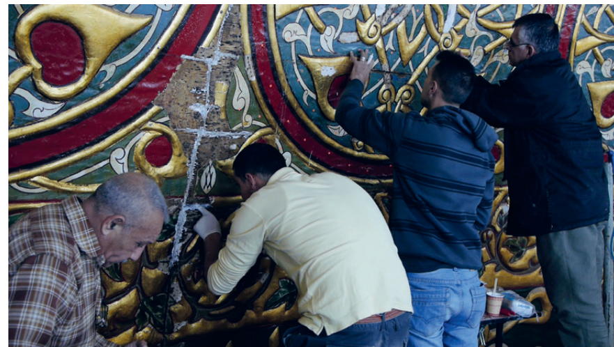
Maeve Brennan, Jerusalem Pink (UK, 2015). Restorers at work on the dome's interior decorations inside the Dome of the Rock.
